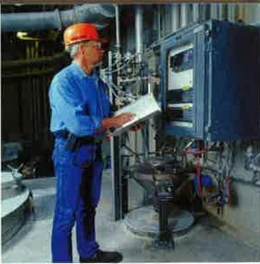
The METTLER TOLEDO Lynx™ controller/display shares an explosion-proof cabinet with two displays used by the Provox system that runs the plant. The Lynx controller zeros the scale before each batch, filters out signal noise caused by vibration, and passes the weight data along to the Provox system.
